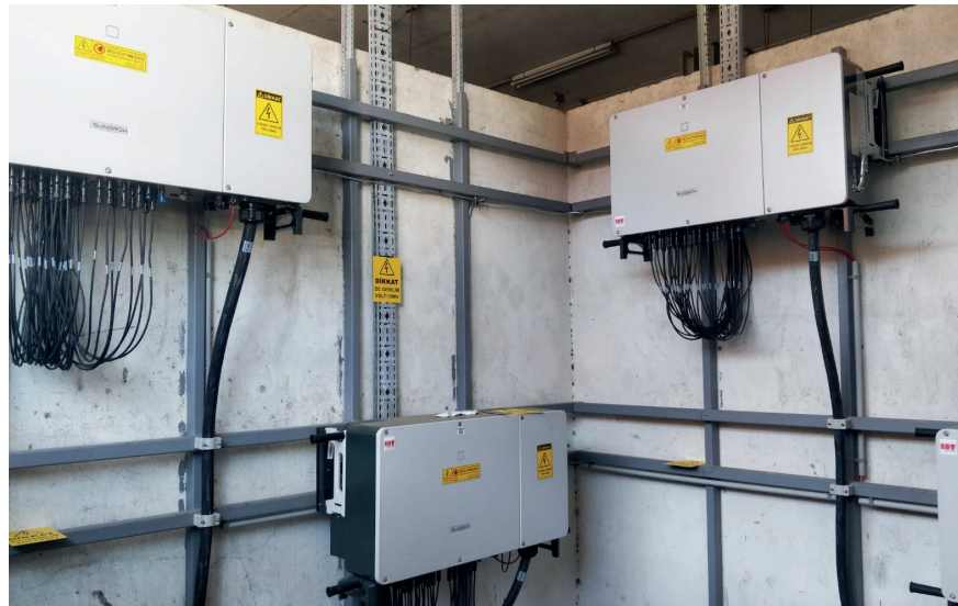
SG110CX inverters have 9 MPPTs for a total of 18 string inputs.
